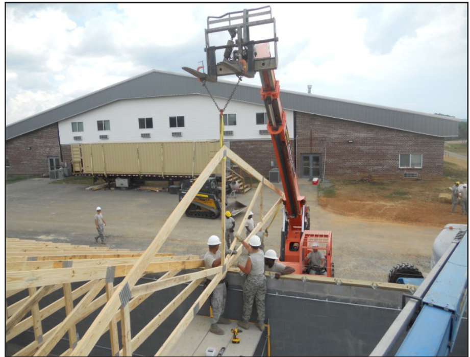
512th Civil Engineer Squadron members install roof trusses on a building at Riverside Christian Academy, a Fayetteville, Tenn., school devastated by tornadoes in April 2011. The Airmen are among the latest in a string of Air Force Reserve Command civil engineer teams to work at the campus. (Courtesy photo)
