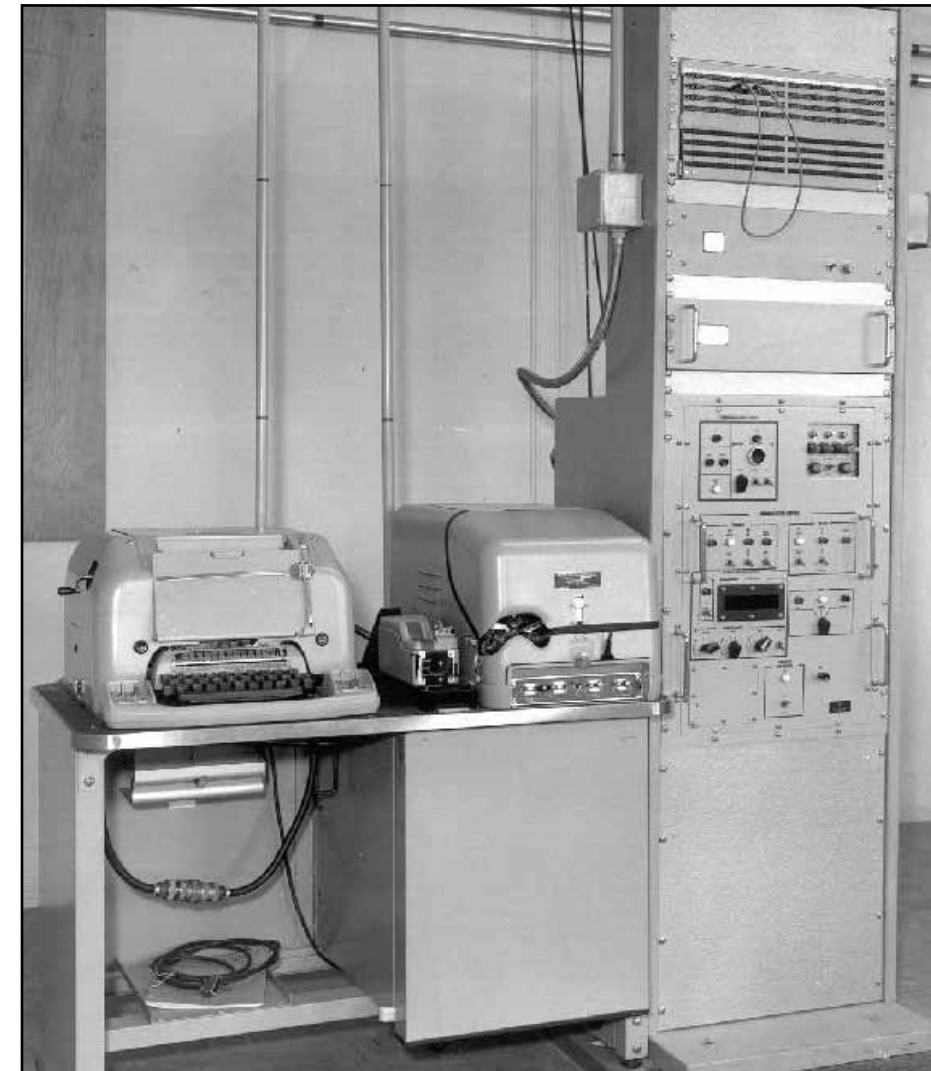
From left to right are an Autodin Mode 5 Terminal, a Kleinschmidt teletype, a tape reperforator including an externally affixed paper tape reader and the Autodin Mode 5 unit in the rack. These are the same types of equipment Al Dutton used when he was assigned to Dover Air Force Base's Communications Center in the 1960s. (Photo courtesy Fort Monmouth Historical Office/ submitted by George Mace)
