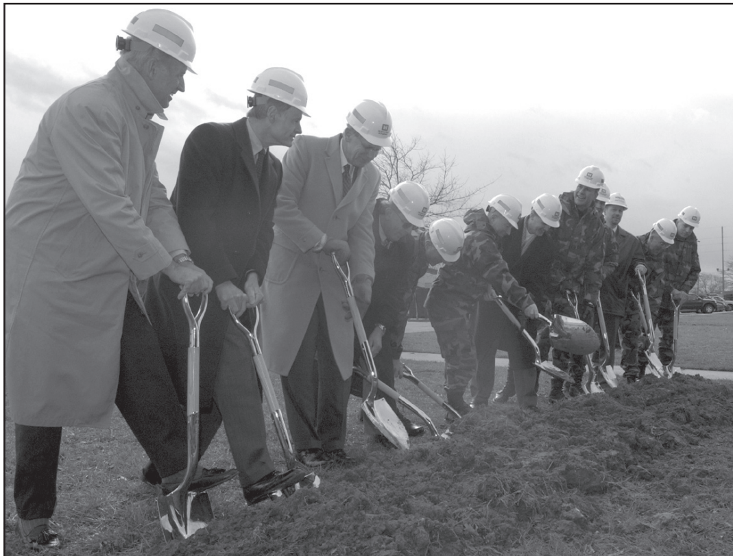
TOP: Lt. Gen. William Welser III, 18th Air Force commander, addresses the Dover Team Dec. 12, 2004, during the ground breaking of Dover's new Super Port. BOTTOM: Delaware U.S. Senators Joseph Biden and Thomas Carper, Delaware U.S. Congressman Michael Castle, General Welser and other dignitaries join Col. Ronald A. Rutland and Col. John I. Pray Jr., 512th and 436th Airlift Wing commanders respectively, in the ground breaking of the base's new aerial port.
